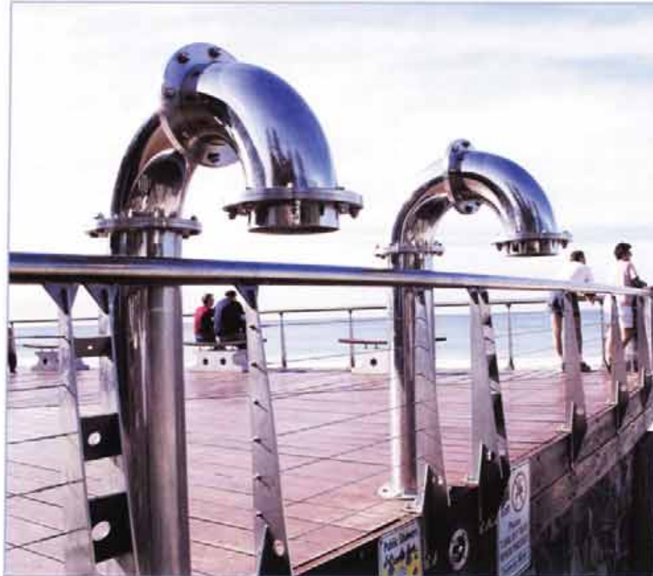
ABOVE: A successful stainless steel installation in a coastal application, with no tea staining
